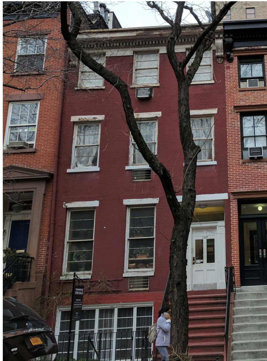
EXISTING FRONT FACADE
