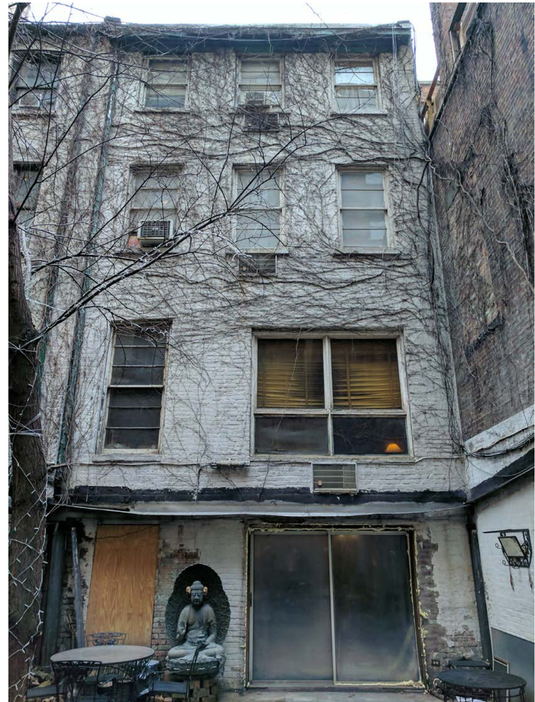
EXISTING REAR FACADE
